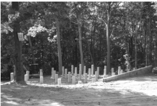
The new foundation is underway.
